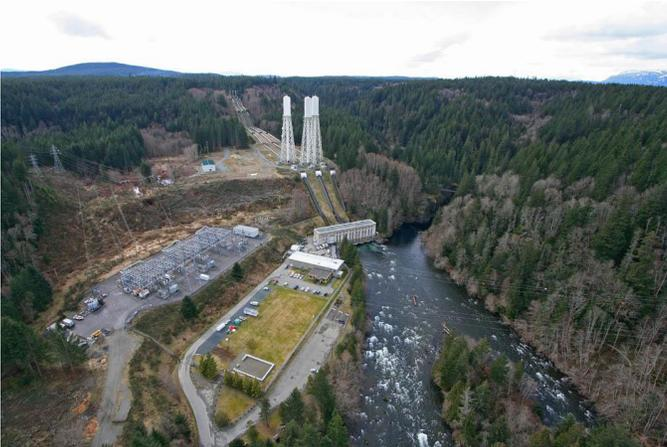
In May 2009, BC Hydro proceeded to undertake a study program for the “John Hart Powerhouse Replacement”, which comprised investigations to replace the current powerhouse, a 62 year old facility requiring upgrading at the John Hart Generating Station (BCHJGS). The site area covers an area of approximately 5,000 m<sup>2</sup>, and the proposed powerhouse has a footprint of approximately 2,660 m<sup>2</sup>, which will transmit foundation loads directly to underlying bedrock strata.
