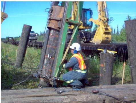
On August 15<sup>th</sup> 2008, GES Geotech completed PDA Testing and a Geotechnical Analysis report to assess the measured pile capacities and the foundation of the CN Rail Bridge at the south of Fort McMurray in Alberta, estimating in 16" (40.7mm) for timber piles diameter.
